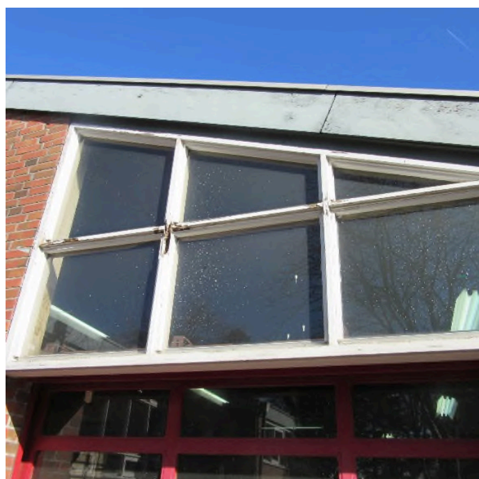
Figure 3 Serious wood rot in almost all frames of the building. Antea Group, 2019.
