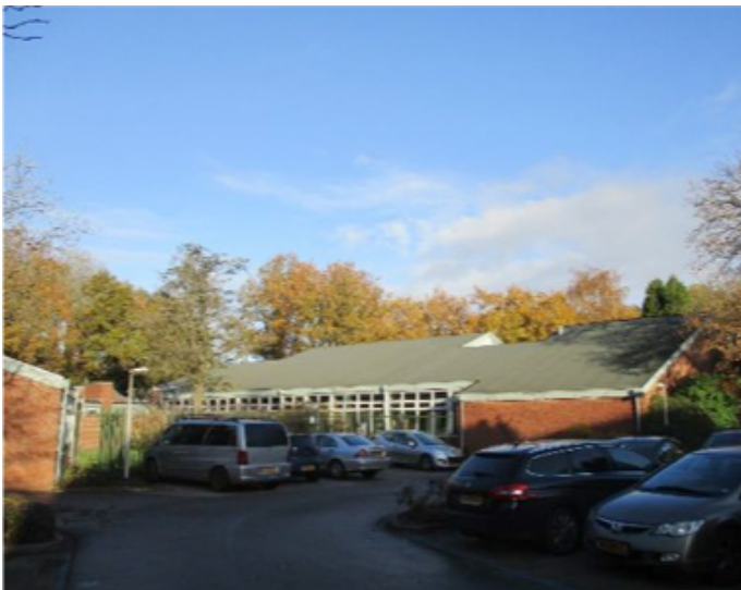
Figure 15 Rear view of the building, Ecocert, 2019.
