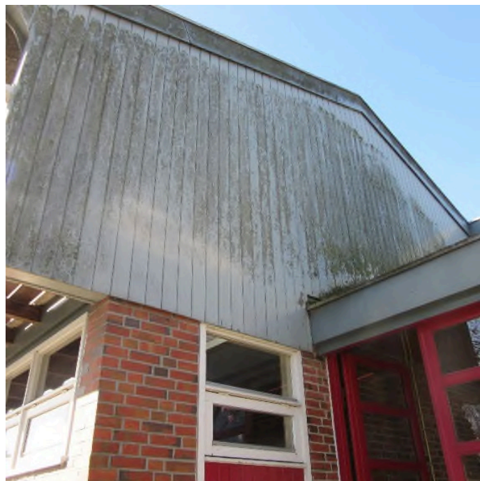
Figure 2 Dirty wooden cladding on the building's facade. Antea Group, 2019.
