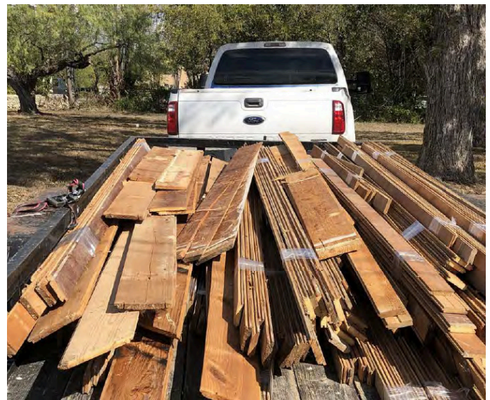
Figure 59 A portion of the reclaimed flooring and shiplap, ready to be transported off site from the San Antonio City's second Certified Deconstruction Contractor Training. Placeconomics, 2021.
