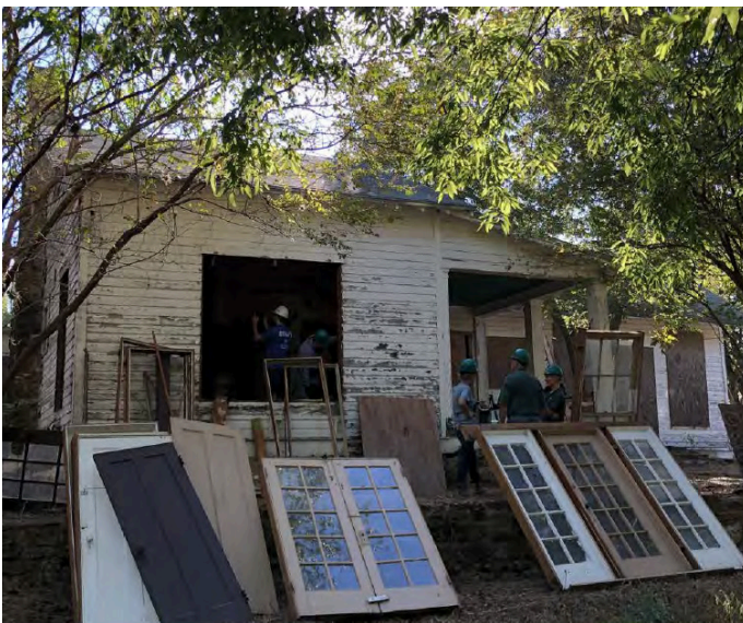
Figure 58 Some of the reclaimed materials demounted during the deconstruction contractor training workshop, City of San Antonio Certified Deconstruction in 2019. Placeconomics, 2021.
