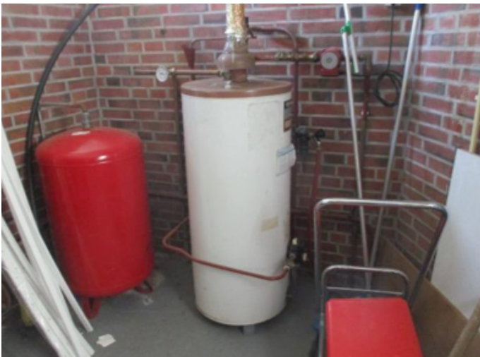
Figure 18 Old water heating equipment currently operating in the building, Syplon Maintenance Plan, 2020.
