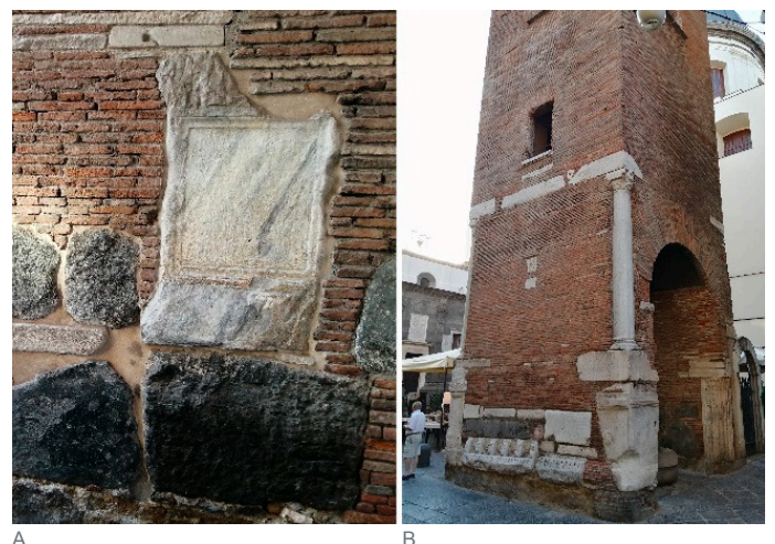
Figure 53 Reused elements in the base (A) and the rear side (B) of the bell tower of Santa Maria Maggiore della Pietrasanta. Bertino et al., 2021 .
