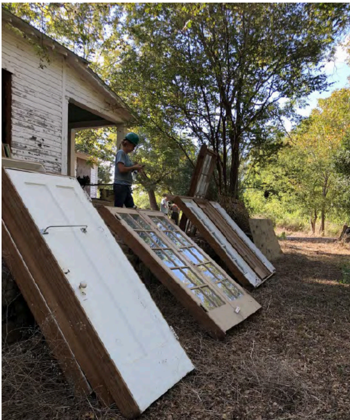
Figure 50 Flooring reclaimed during a City of San Antonio Certified Deconstruction Contractor Training, set aside for de-nailing by participants. Placeeconomics, 2021.
