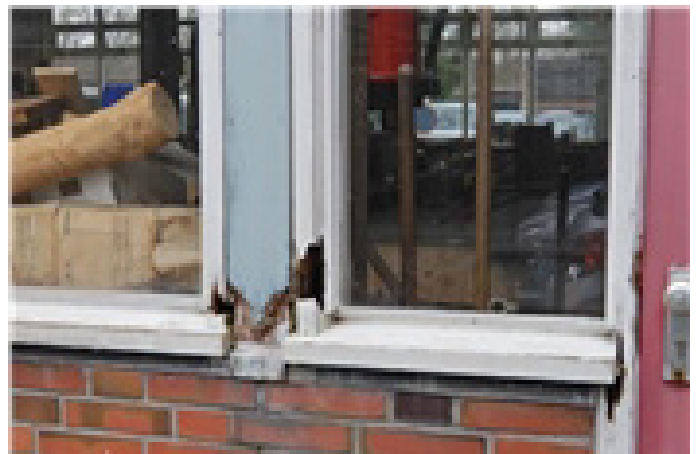
Figure 19 Visible damages on window frames, Syplon Maintenance Plan, 2020.
