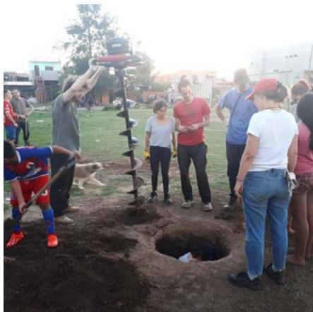
[4], [5] Collaborative Construction Project between Universities (FADU-UBA, UNSAM) and La Biblioteca Popular, October 2019
