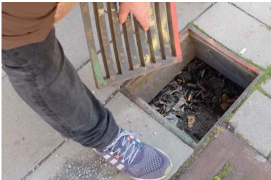
Fig. 4.06 Air and stormwater inlet
