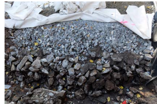
Fig. 4.11 Structural soil and aerated bearing layer
