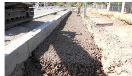
Fig. 4.16 Crushed rocks with tackifier and planting soil
