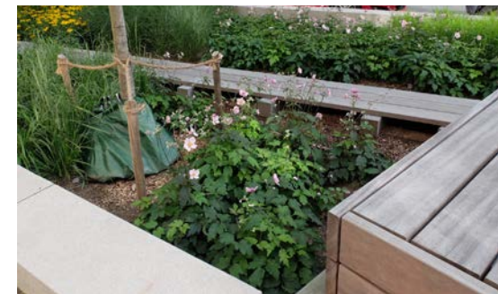
Fig. 4.03 Decentralized Stormwater Management (Infiltration Raindarden) in Norra Djurgårdsstaden, Stockholm
