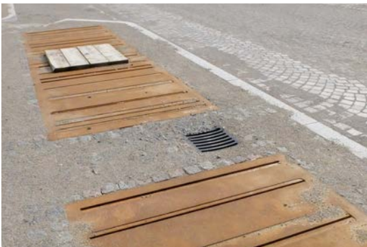
Fig. 4.08 Preparation of tree pits in construction process
