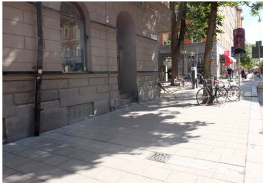
Fig. 4.12 Stormwater interception (roof and sidewalk)
