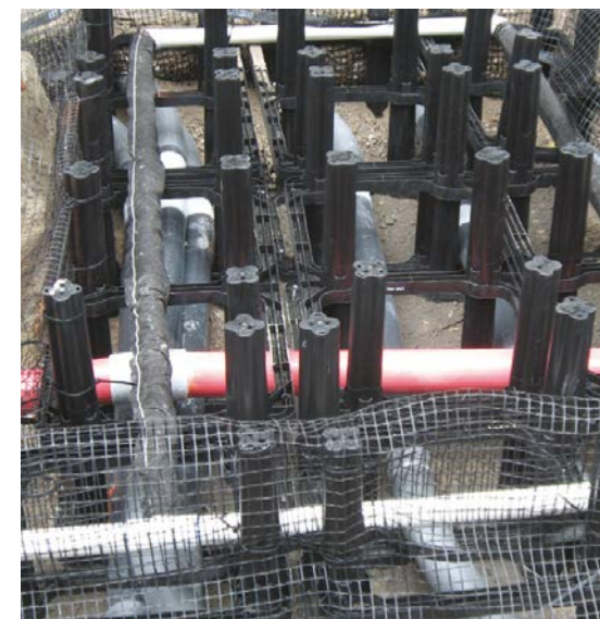
Fig. 4.27 Silva Cells with planting soil and pipes
