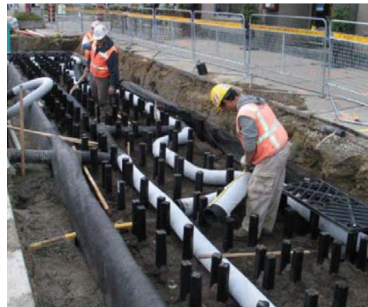
Fig. 4.26 Construction process of Silva Cells
