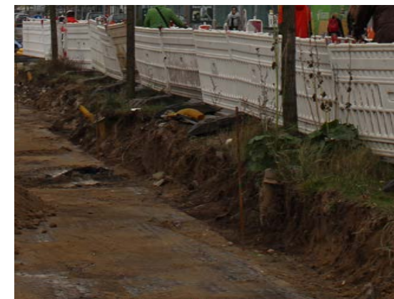
Fig. 5.03 Construction excavation around root ball
