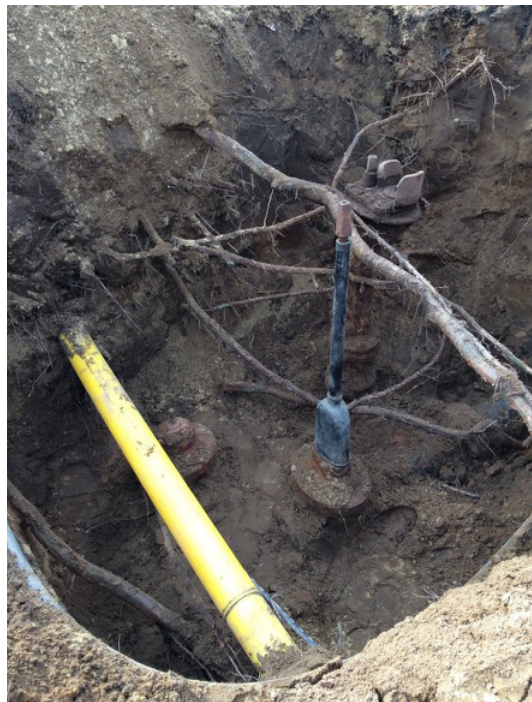
Fig. 5.02 Excavation around tree roots
