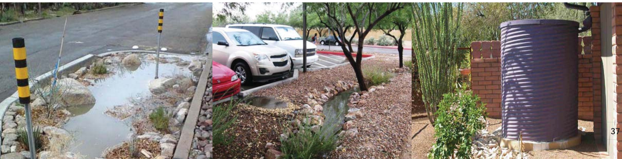
Figure.22: Active & passive rainwater harvesting in Tucson,AZ
