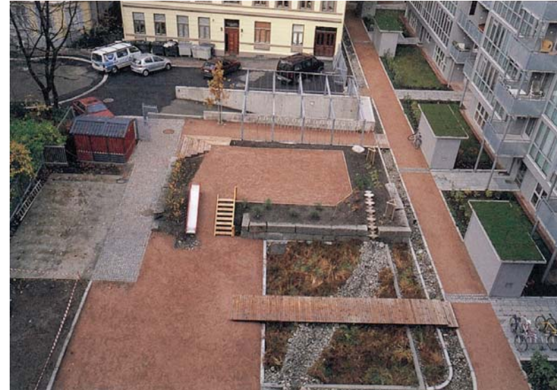
Figure.61: Decentralized greywater treatment in urban areas - Klosterenga, OSLO, Norway
