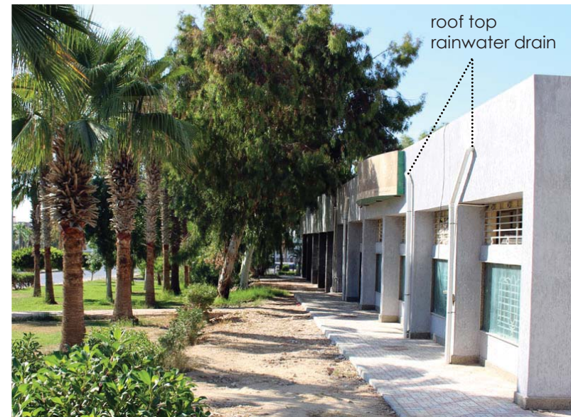
Figure.45: Roof top pipes drain rainwater to the sewage, but not benefitting the adjacent green space
