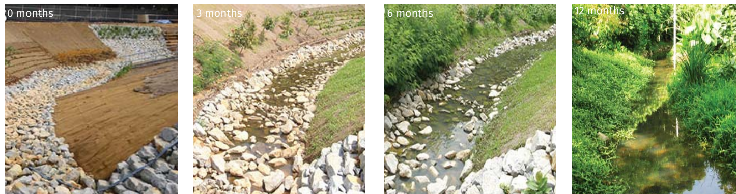
Figure 44. Progress of Soil Bio-engineering over a one-year period. Photo: Ramboll Studio Dreiseitl. Taken from: (ASLA, 2017)
