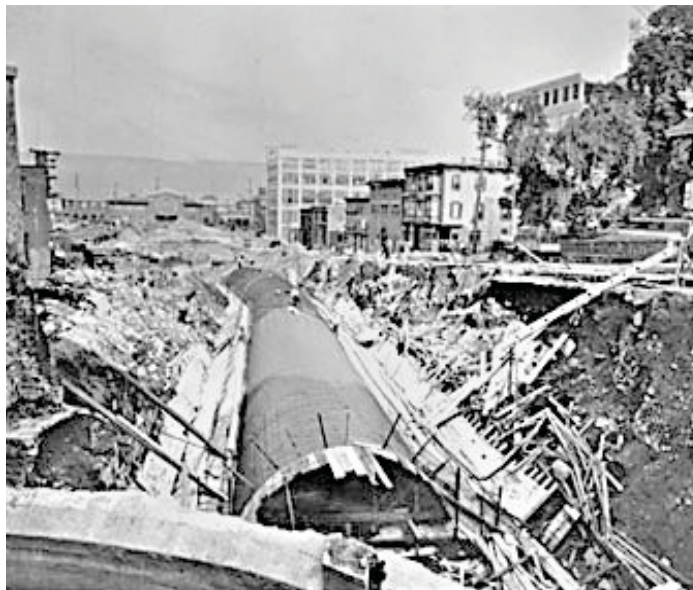
Figure 33. Construction of the Underground Flume through which the Saw Mill Flows since 1922. Taken from: (Saw Mill River Coalition, 2017)
