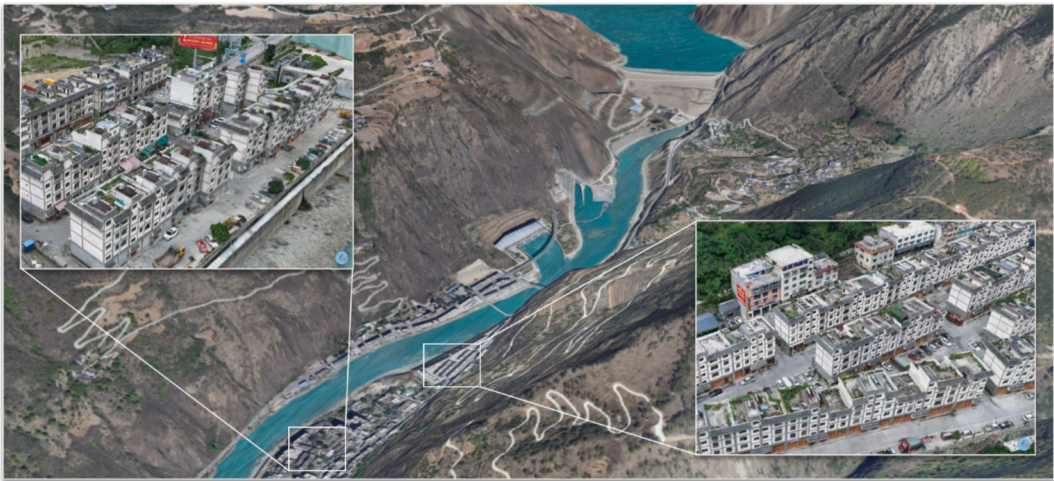
Fig. 17. 3D representation of large-scale environment landscape surrounding the bridge construction.
