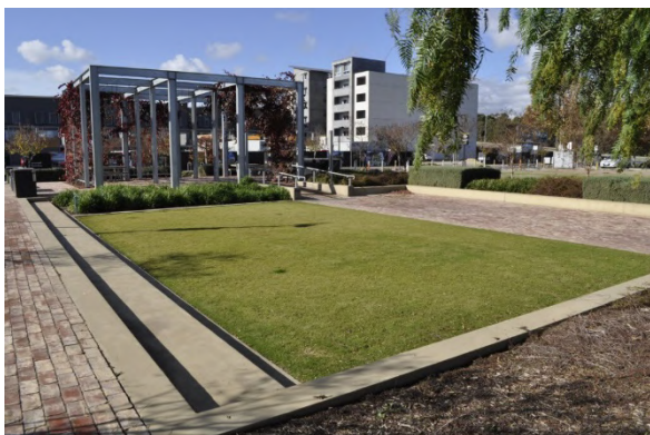
Fig. 3-11: A multifunctional basin for stormwater detention and recreational use in Adelaide, Australia (Water Sensitive SA, 2023).
