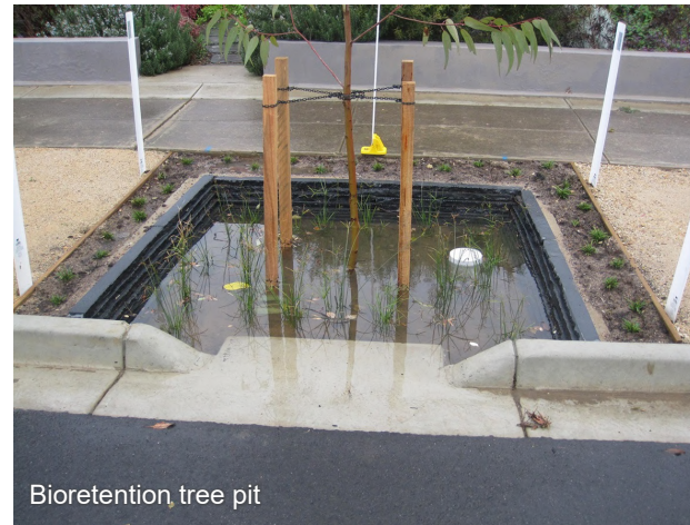
Fig. 3-22: Example types of bioretention systems showing their adaptability to various scales and urban settings (Photos: Water Sensitive SA, 2023)
