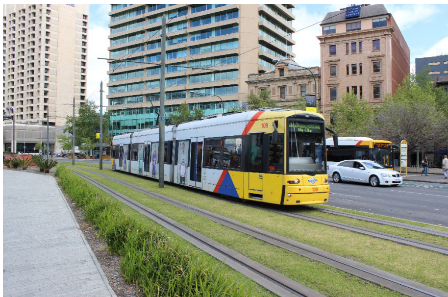
Fig. 3-41: Adelaide green tram track at Victoria Square (Photo: Philip Mallis, 2015)
