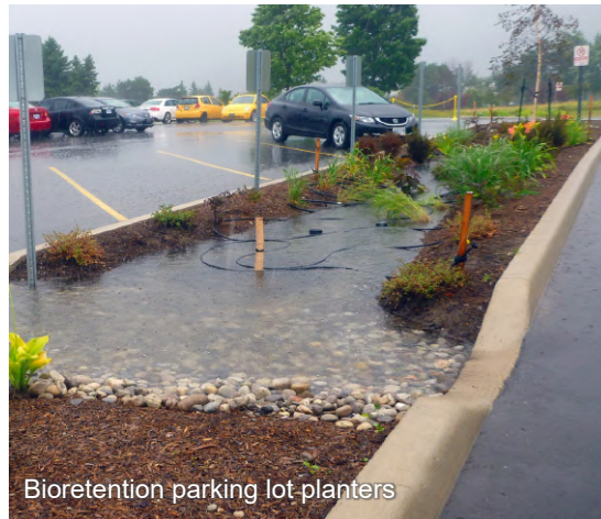
Fig. 3-22: Example types of bioretention systems showing their adaptability to various scales and urban settings (Photos: Water Sensitive SA, 2023)
