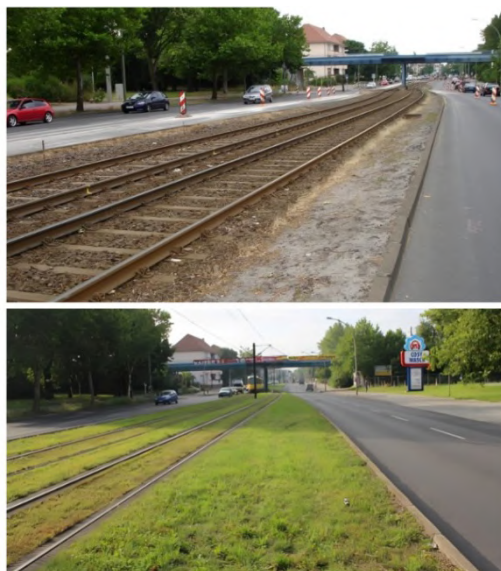
Fig. 5-33: Ballasted tracks before and after greening in Berlin (Image: Dreger, BVG and Schreiter, IASP)
