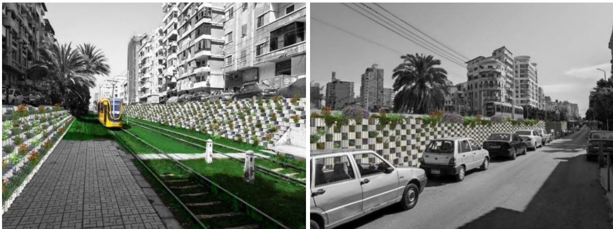
Fig. 5-37: Further variations of modular blocks system for sloped retaining wall in lower track, and strait wall in upper track (Illustration by Mohamed Elfouly on photos by author)
