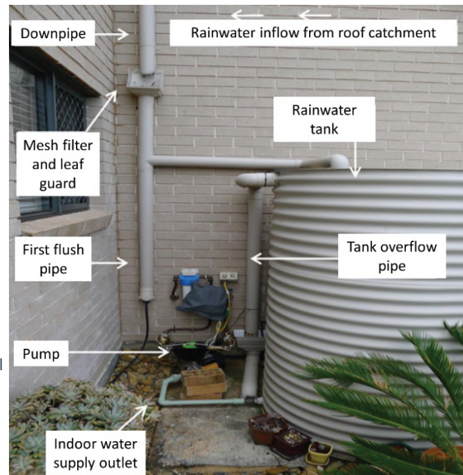
Fig. 3-28: Typical end-user connections for using rainwater in households and an example of a typical residential rainwater system setup with an external pump in Queensland, Australia (Sharma, 2015)
